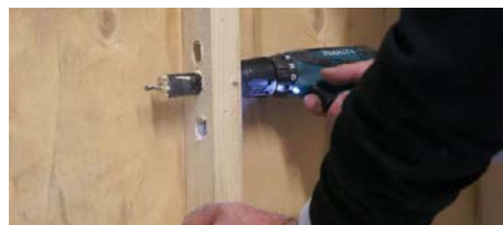
1. Drill holes in the structure for pipes
