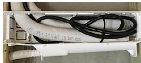
7. Insert wiring and connect drain
