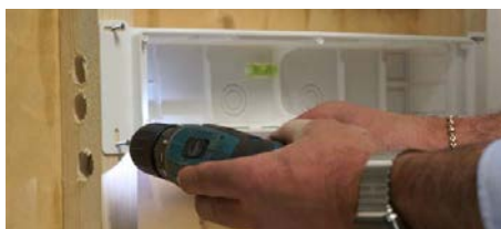
5. Fix box to the structure using screws
