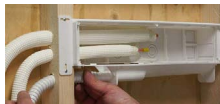
6. Insert pipes and drain hose
