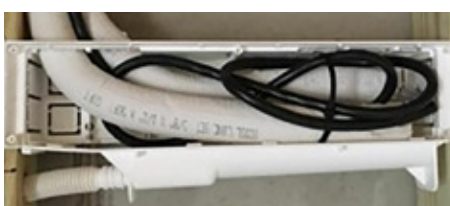
7. Insert wiring and connect drain
