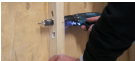
1. Drill holes in the structure for pipes
