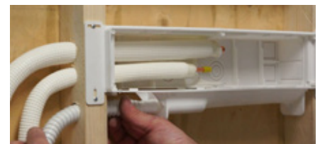
6. Insert pipes and drain hose
