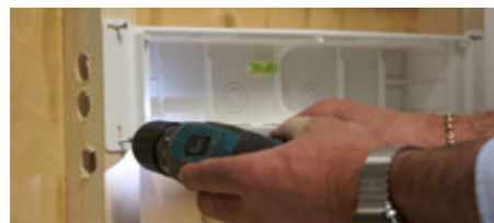
5. Fix box to the structure using screws
